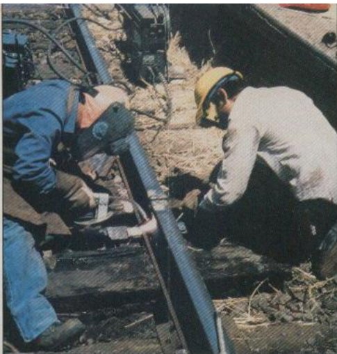
Fig. 1—The bottom flange of the rail is joined with a conventional self-shielded flux cored electrode.
